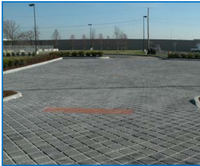
Permeable pavement parking lot with underground storage.
